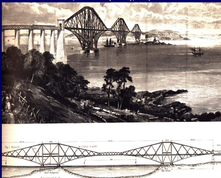
most Firth of Forth , Škotska (1890), raspon L=521\text{m}
