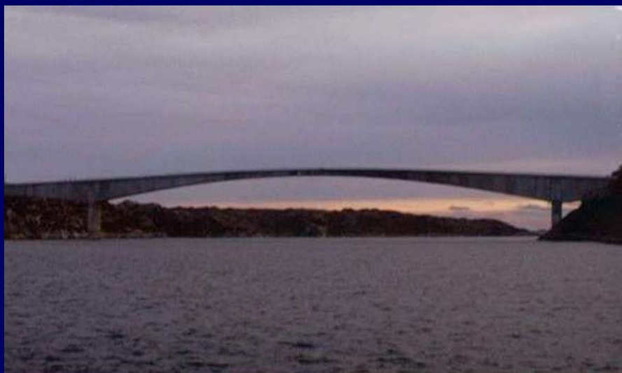
most Stolmasundet , Norveška (1998), raspon L=301\text{m}
