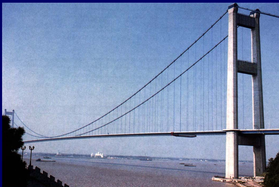
most Jiangyin , Kina (1998), raspon L=1.385\text{m}
