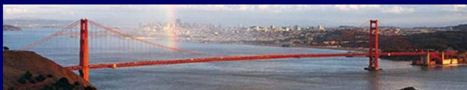
most Golden Gate , San Francisco (1937), raspon L=1.280\text{m}
