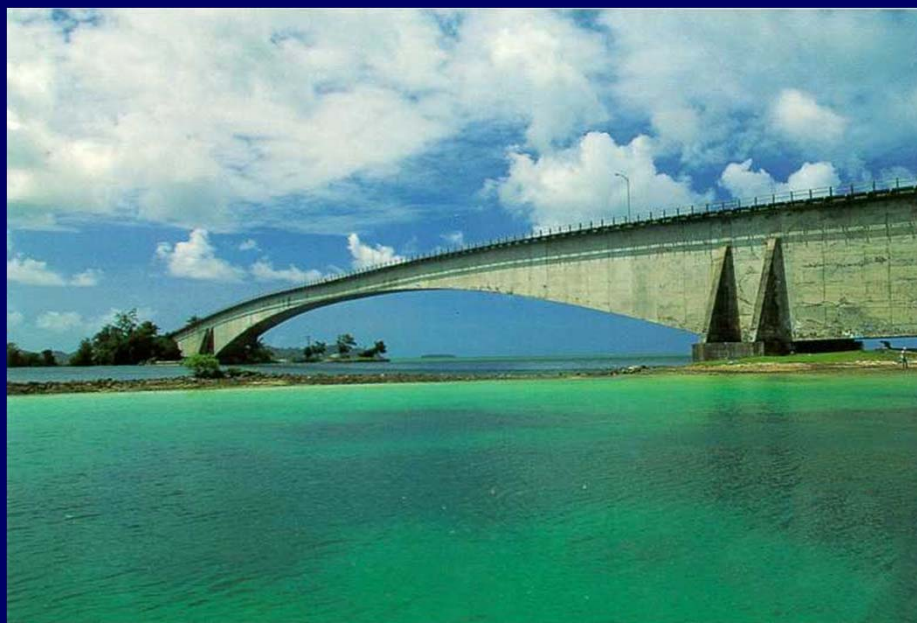
most Koror-Babelhuap u Palau (1977), raspon L=241\text{m} , srušio se 1996.g.
