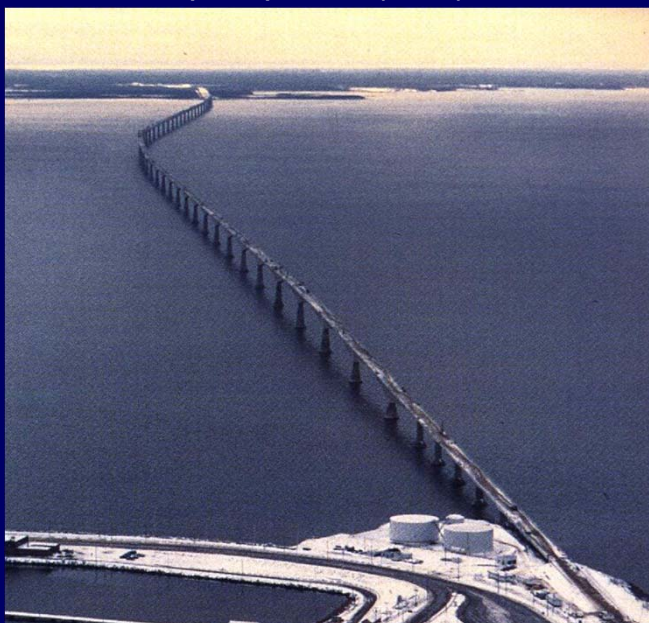
most Northumberland (Confederation Bridge) , Kanada (1997), 43 raspona po 250m
