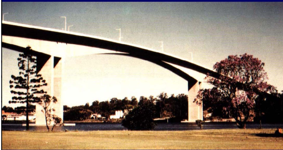
most Gateway , Australija (1986), raspon L=260\text{m}
